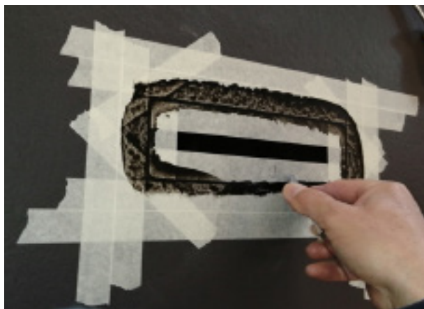
Fig.10 - How to protect the top from the silicone phase and subsequent cleaning / uniformity of the silicone
